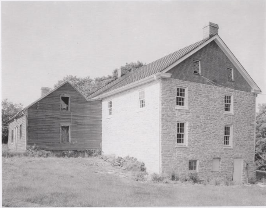
South Gable – Showing original front
