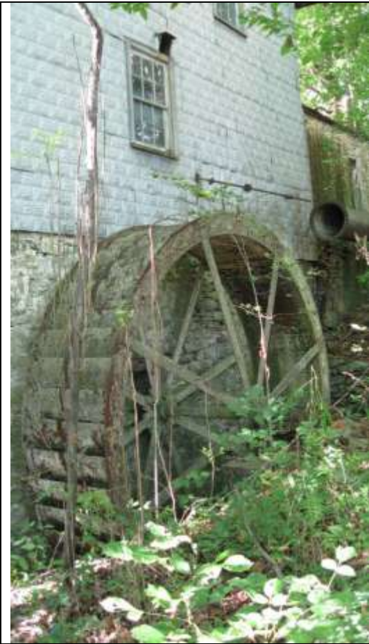
Figure 3. Feagans' Mill from the north showing Fitz Water Wheel manufactured in Martinsburg, West Virginia. WV_Jefferson_County_Feagans'_Mill_0003
