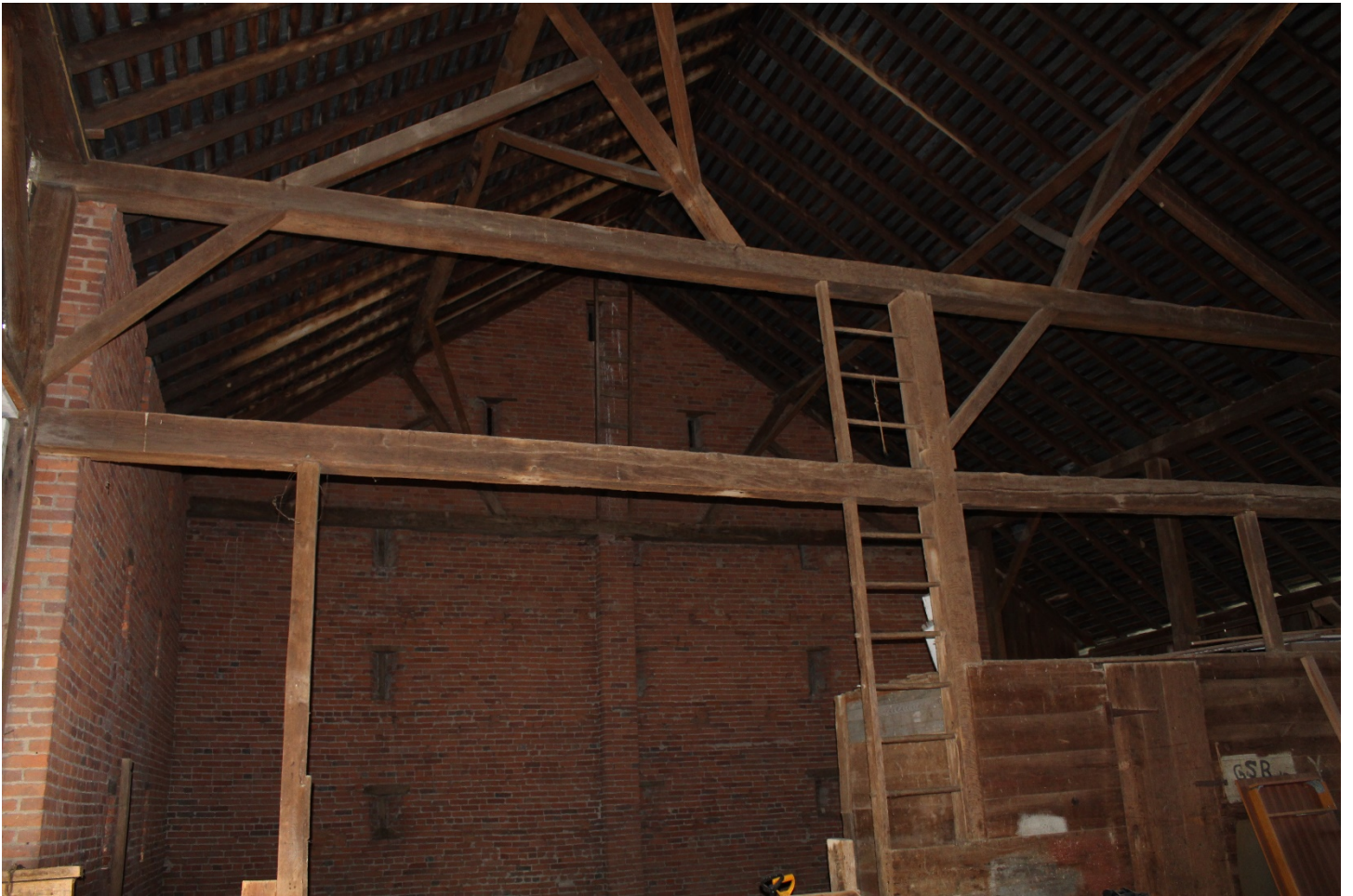
Image showing rafter details and the original southern gable end
