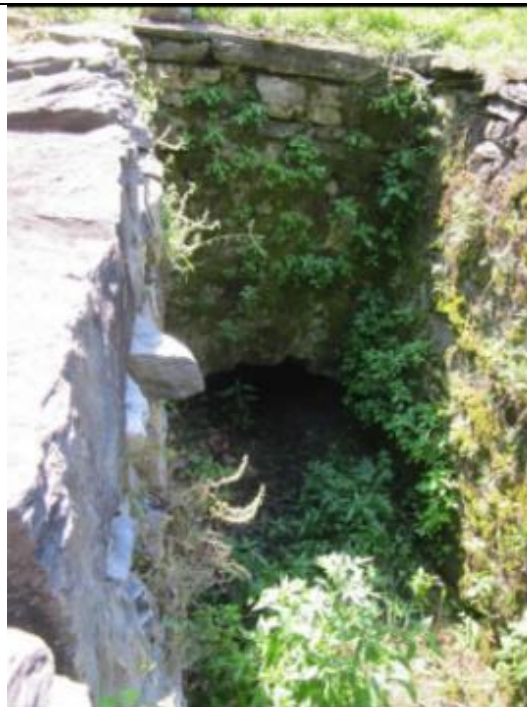
Photo 12. Weirick and Weller Waterwheel, tailrace, East end entry to a stone tunnel/culvert that extends beneath Kabletown Road, view ESE.
