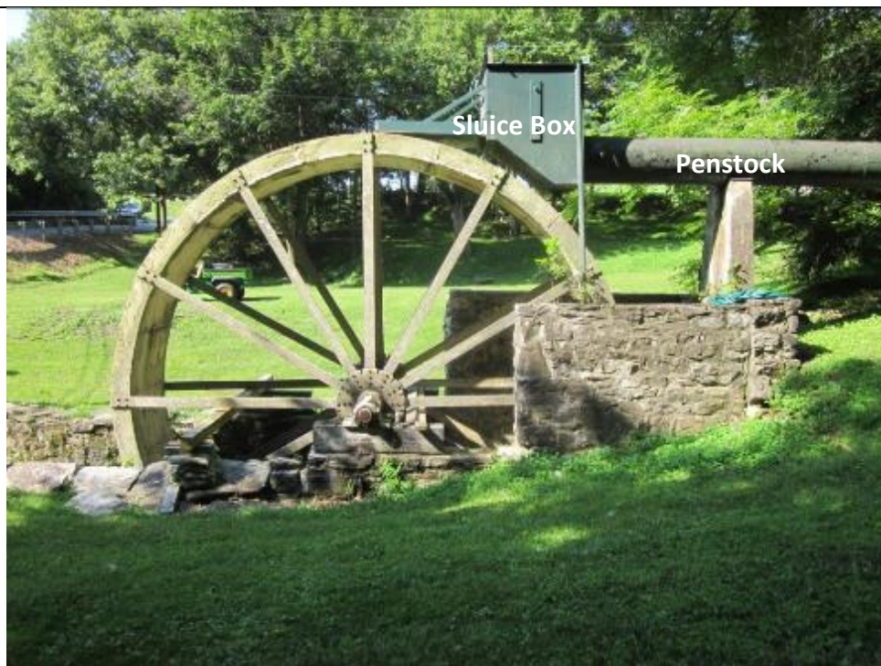
Photo 10. Weirick and Weller Waterwheel, north side of wheel, with Sluice Box and Penstock., view SE.
