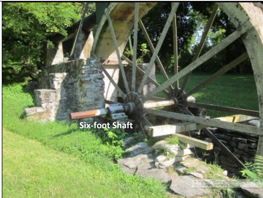
Photo 11. Weirick and Weller Waterwheel, (south side), highlighting the six-foot shaft that would have connected to the milling equipment, view N.
