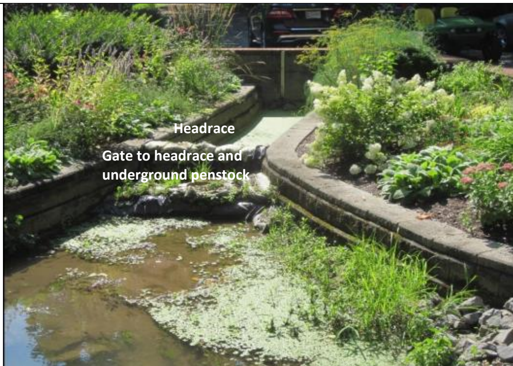
Photo 6. Headrace with gate to underground penstock. View East.
