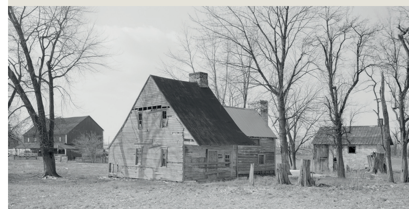
1933 Photos of the Peter Burr House from the Historic American Building Survey, courtesy of the Library of Congress
