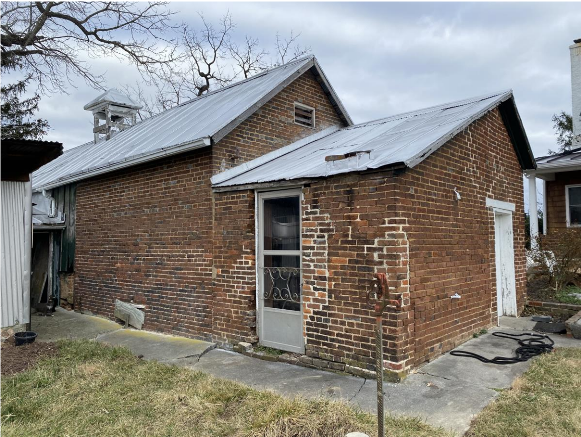
Photo 11: Southwest view of summer kitchen and smokehouse.
