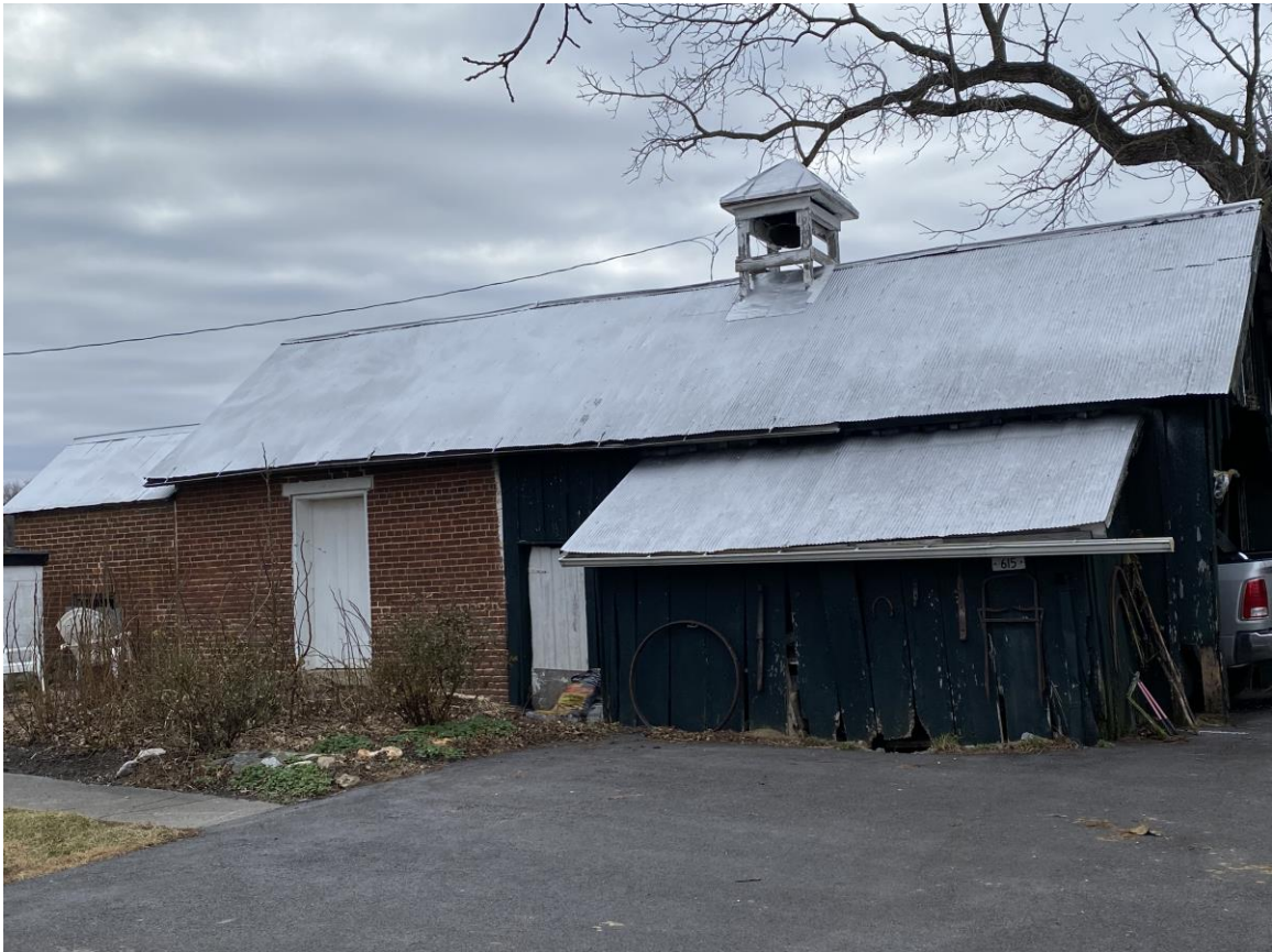
Photo 10: East view of smokehouse, kitchen, school, and garage addition.
