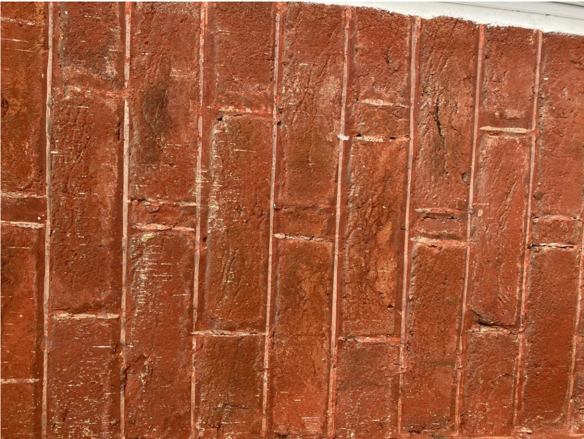
Photo 7: Preserved penciling of joints on brickwork under side porch.
