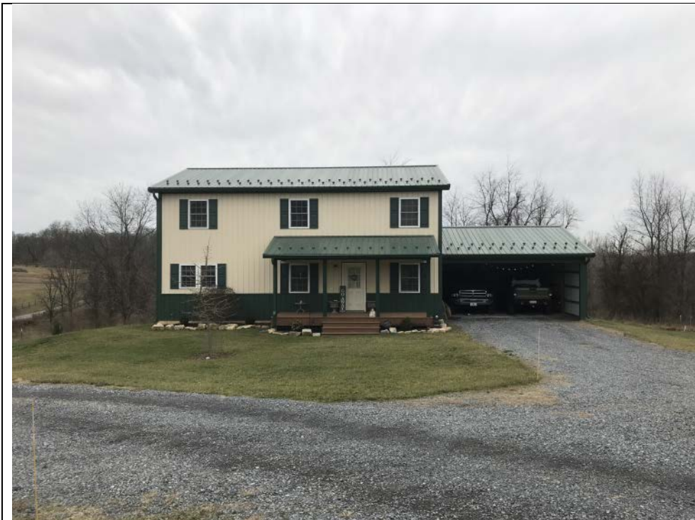
WV_Jefferson County_Woodbyrne_0005. Tenant house, front façade, view to west.
